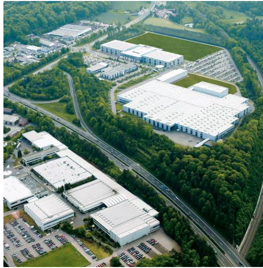
Festo Factory and Customer Service Center, St. Ingbert
